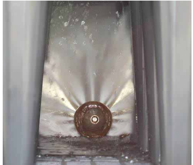
FIG. 3 High pressure jetting possible
