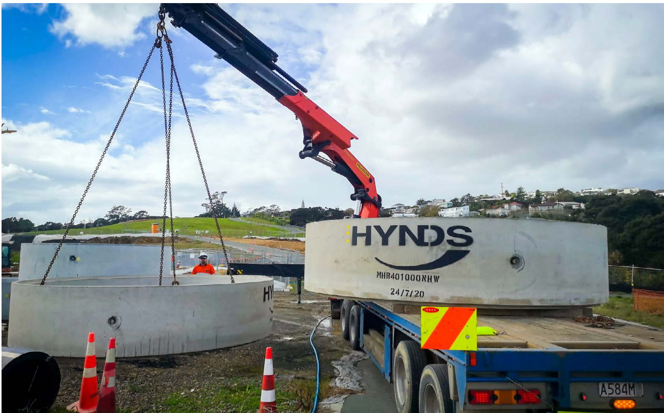
FIG. 1 Photo of 4m Manhole on site.
