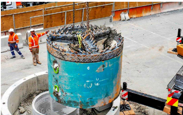
FIG. 4 Drilling head for TBM
