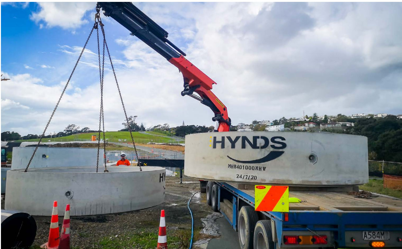
FIG. 1 Photo of 4m Manhole on site.
