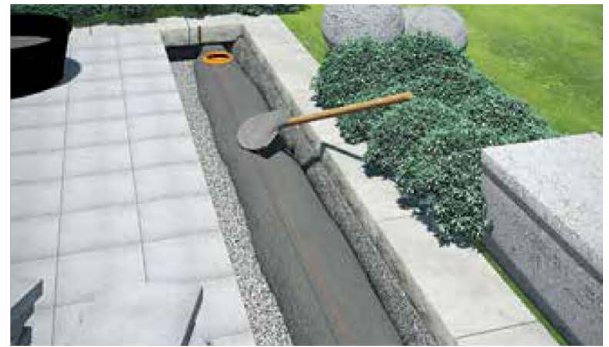
Fill with concrete and compress to foundation.
