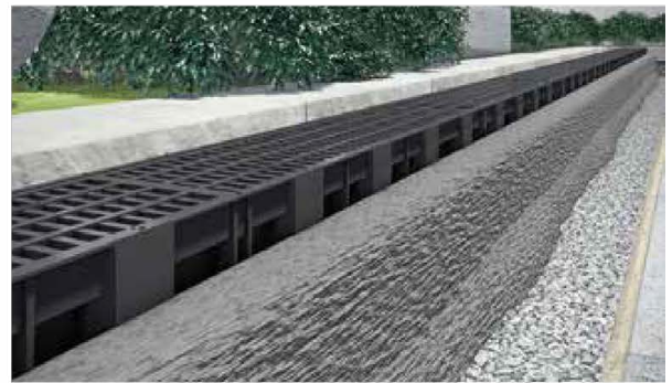
Haunch the concrete.
