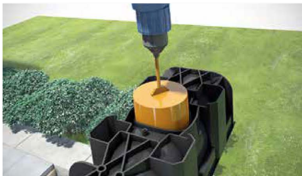
Produce connection openings.
