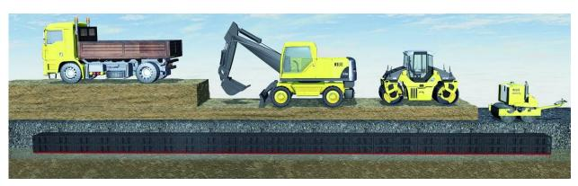
Various construction machinery may be used to fill the excavation. Given the additional dynamic loads they cause, compression equipment must not be driven directly over the EcoBloc Inspect smart system and compression equipment with activated vibration motors must not be taken over the area.
