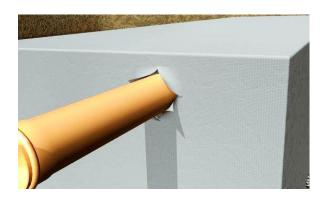
The vents needed are produced in the same way. The vertically aligned vents can be produced on the horizontal drill surface using a 90° bend (plastic pipe bend).
